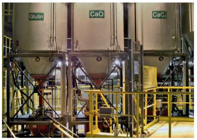
Powder injection silos, Salzgitter, single ladle furnace
