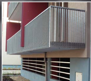
GRATES AS BALCONY RAILING
